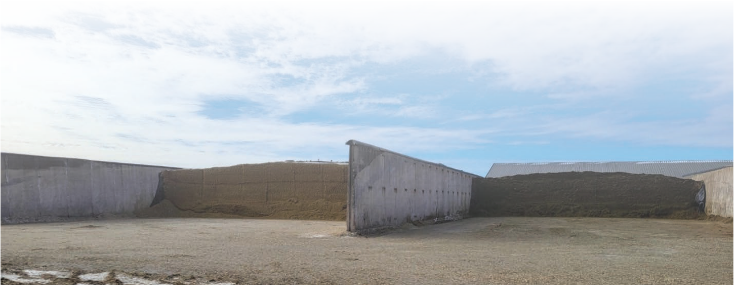
Haylage and Corn Silage bunker at Clark Co. Line
