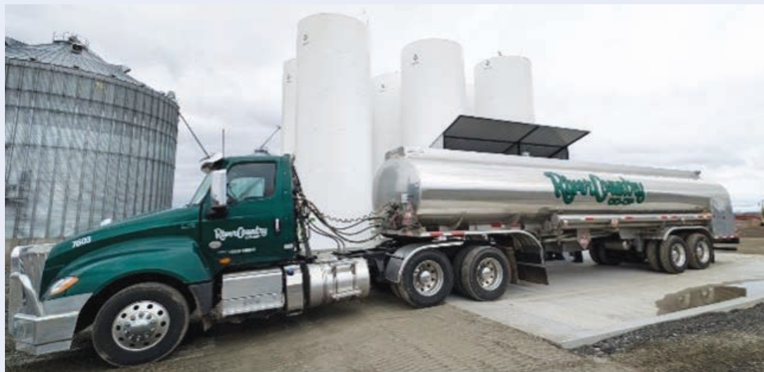
New fuel depot in Athens, WI
